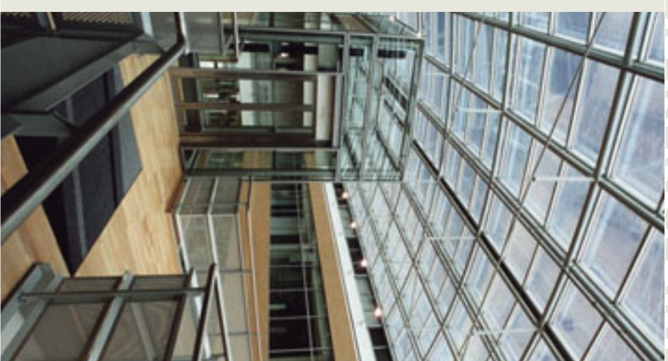
Procter & Gamble, Schwalbach 2000 600 m 2 of micro louvers Architects: Aukett & Heese, Berlin Lighting consultants: von Kardorff, Berlin
