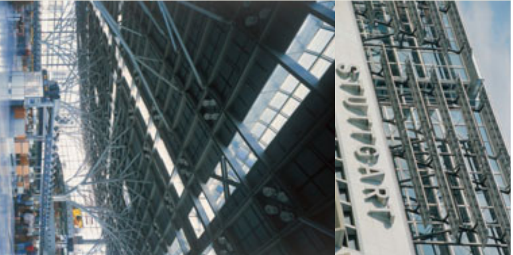
Stuttgart Airport 1989 600 m 2 of prism systems Architects: Von Gerkan, Marg & Partner, Hamburg Lighting consultants: Bartenbach Lichtlabor, Innsbruck
