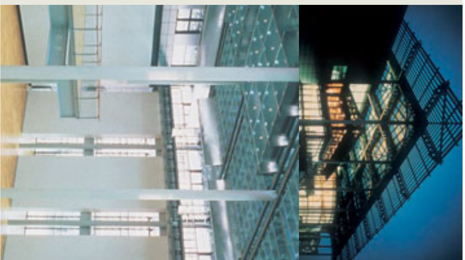
Wolfsburg Art Museum 1992 1500 m 2 of micro louvers in pyramid roofing Architects: Schwieger & Partner, Hamburg Lighting consultants: Bartenbach Lichtlabor, Innsbruck
