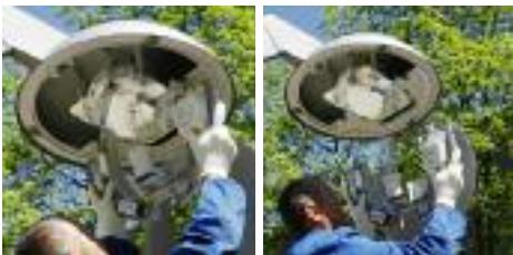
Complete replacement: the gear tray can be removed and replaced.
